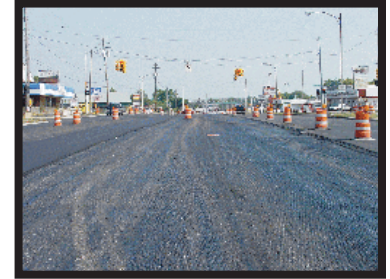
Interlayer Construction Over Milled Surface
