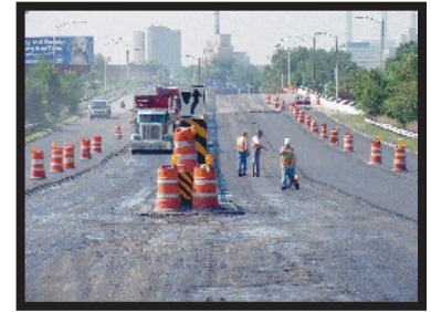
Interlayer Construction Over Milled Surface
