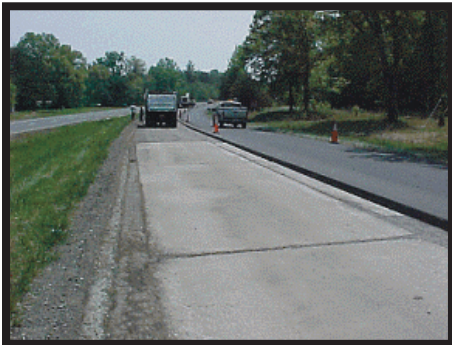
Surface condition after milling
