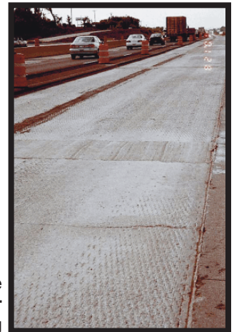
Surface condition after milling
