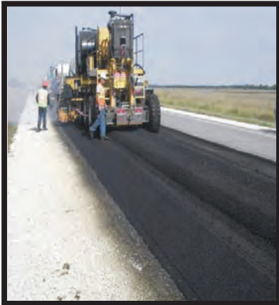
Restore® Hot In-Place Recycling Process
