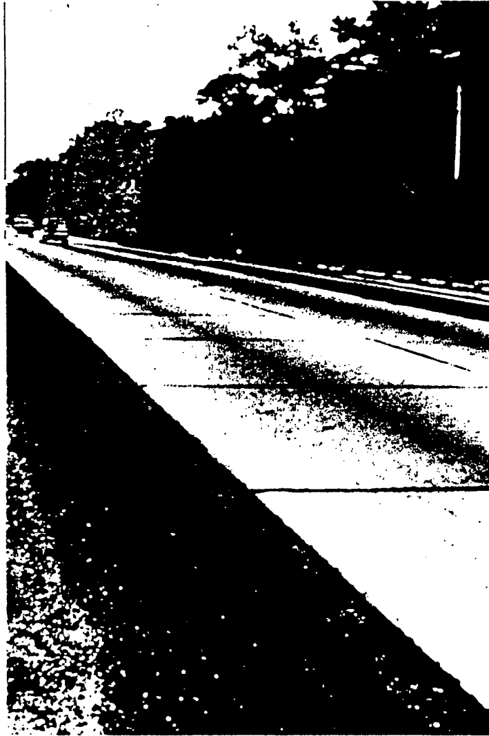
Figure 1 - Portland cement pavement prior to NOVACHIP overlay
