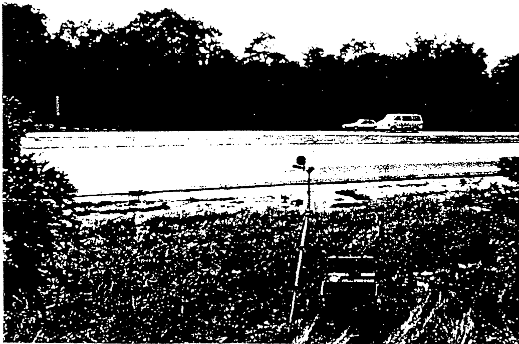
Figure 9 - Test site at MP 83.18 ready for measurements before paving
