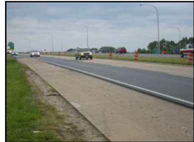
Delaware SR-1 with BondTekk™ CR crack resistant overlay
