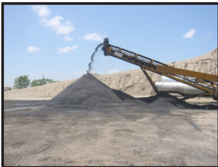
Sedgwick County warm mix from pug mill discharge
