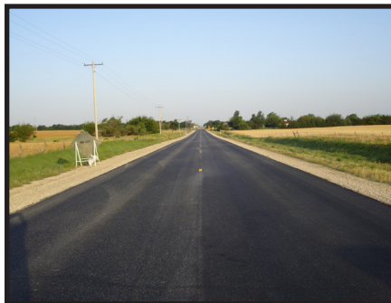
Finished Bonded BM-1 Test Sections
