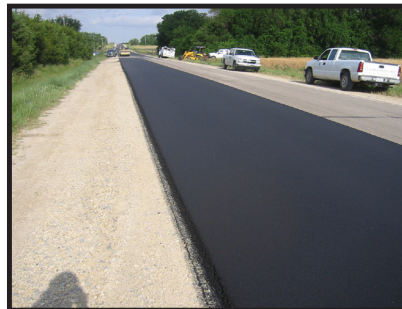
Bonded BM-1 Test Sections just after placement
